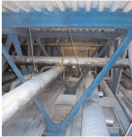
Primed Fireproofing using Fibertech F-50 penetrating primer
