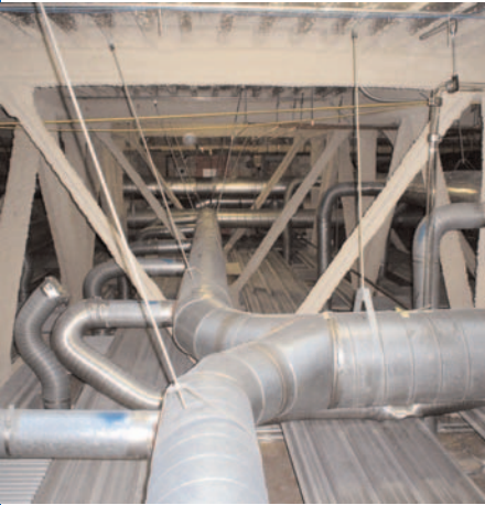
Asbestos fireproofing before Encasement
