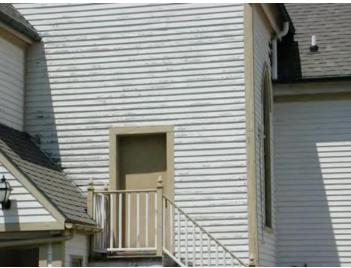
**The Solution:** The ECI FiberTech Encasement System was chosen. The contractor applied one coat of the F-50 Penetrating Stabilizer Primer followed by two coats of the F-51 Sealer Coat. This provided the church with a waterproof coating system that will last for at least 20 years.
