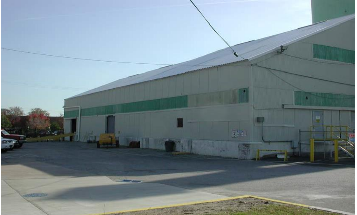
The F-50 Penetrating Stabilizer Primer was allowed to dry for 24 hours before two coats of the F-51 Sealer Coat were applied.
