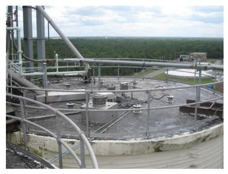
**The Solution:** The FiberTech waterproofing membrane system was chosen due to its long term effectiveness, ease of installation, and cost effectiveness. One coat of the F-50 Penetrating Stabilizer primer followed by one coat of the F-51 Sealer Coat was applied to each of the silos.
