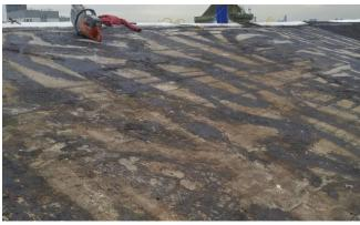
The areas were then scrim coated with our Poly Mesh Scrim Fabric and FiberTech F-50 Penetrating Stabilizer Primer. The primer was allowed to dry and was then coated with two coats of our FiberTech F-51 Roof Sealer Coat. The overall success of the project has led to additional roof applications at the prison.
