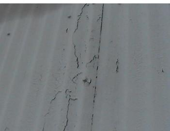
**The Solution:** The ECI Encasement system was chosen. A test patch of the system was provided prior to the start of the project. One coat of the F-50 Penetrating Stabilizer was applied, followed by two coats of the F-51 Sealer Coat. This provided the owner with the system they were looking for.
